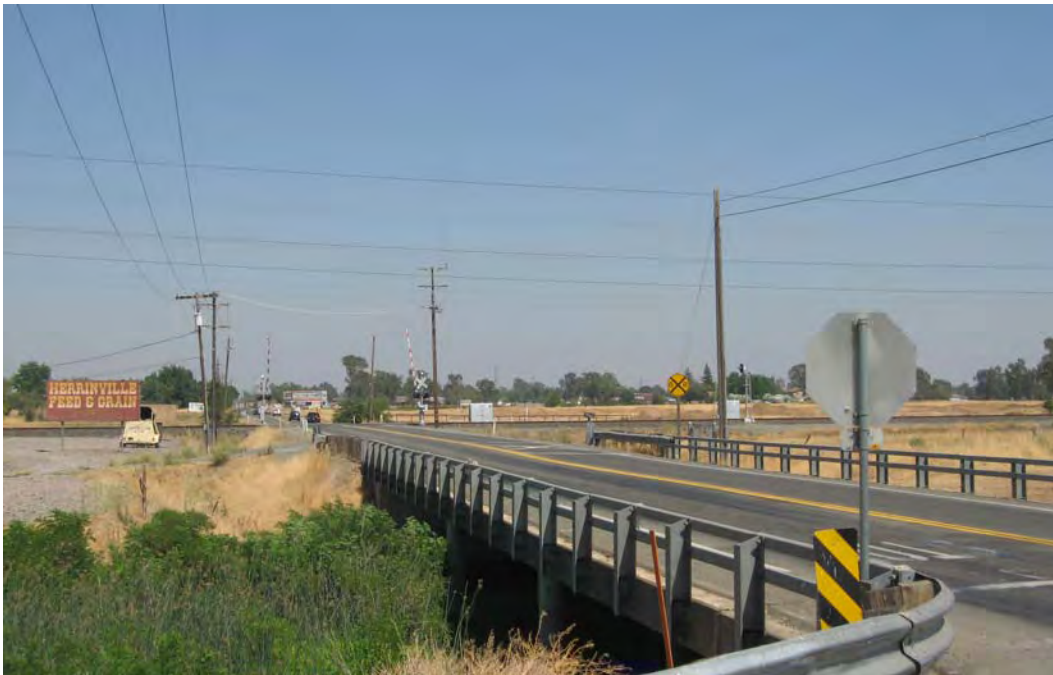
Viewpoint 10. View from the intersection of Natomas Road and Riego Road, looking east along Riego Road at off-site bridge over East Canal, power lines, railroad crossing, commercial structures, and trees. (Photograph taken by EDAW in 2008)
