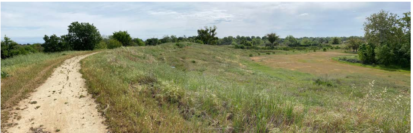
Social trail along the top of the old levee in the Shanghai Bend area
