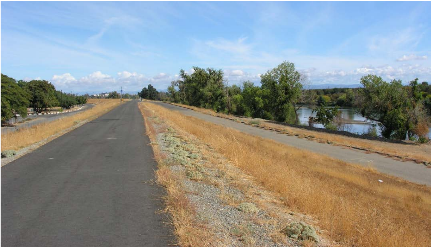
Current bike path on levee top looking north to Marysville
