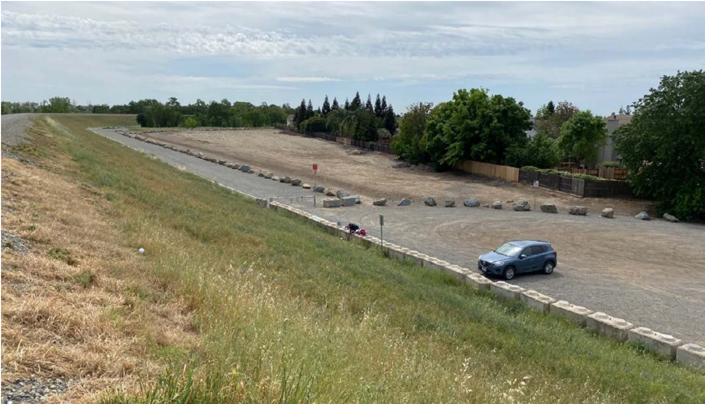
Existing parking area at east end of Shanghai Bend Road
