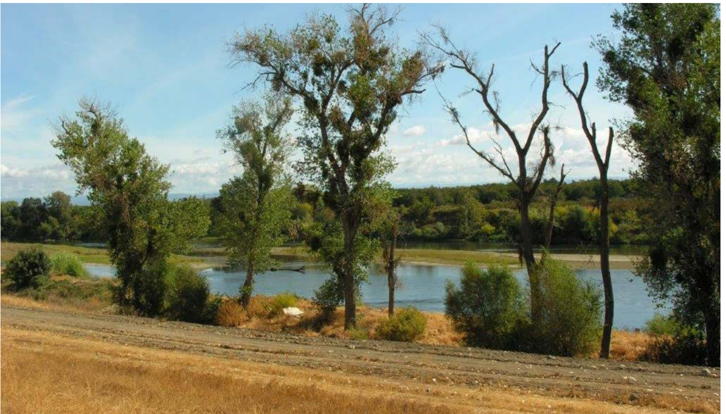
View from levee top towards river
