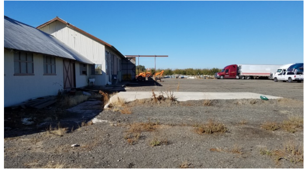
Photograph 8. Large workshop and graveled parking lot within the developed/ornamental portion of the Project site (facing west). Taken on October 18, 2016.
